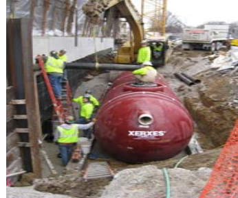
The reclaimed water system collects storm water before distributing to the toilets and urinals.
